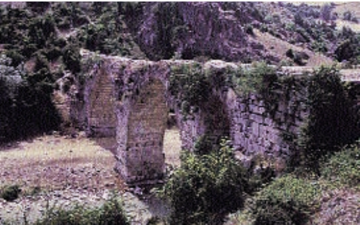
Havza Kurt bridge
