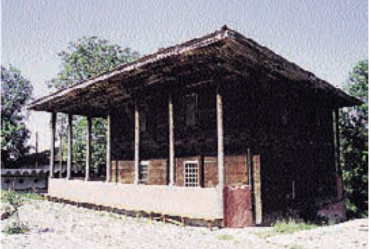
Bekdemir village mosque
