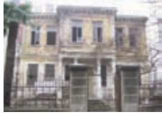
Cemaatoğlu House: This house was left by a Greek called Cemaatoğlu. It is a two-storey masonry structure built on a basement.
